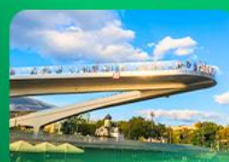
Floating Bridge Moscow
